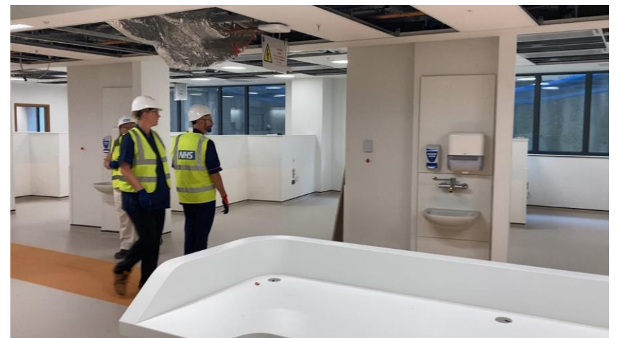
New Discharge Lounge
